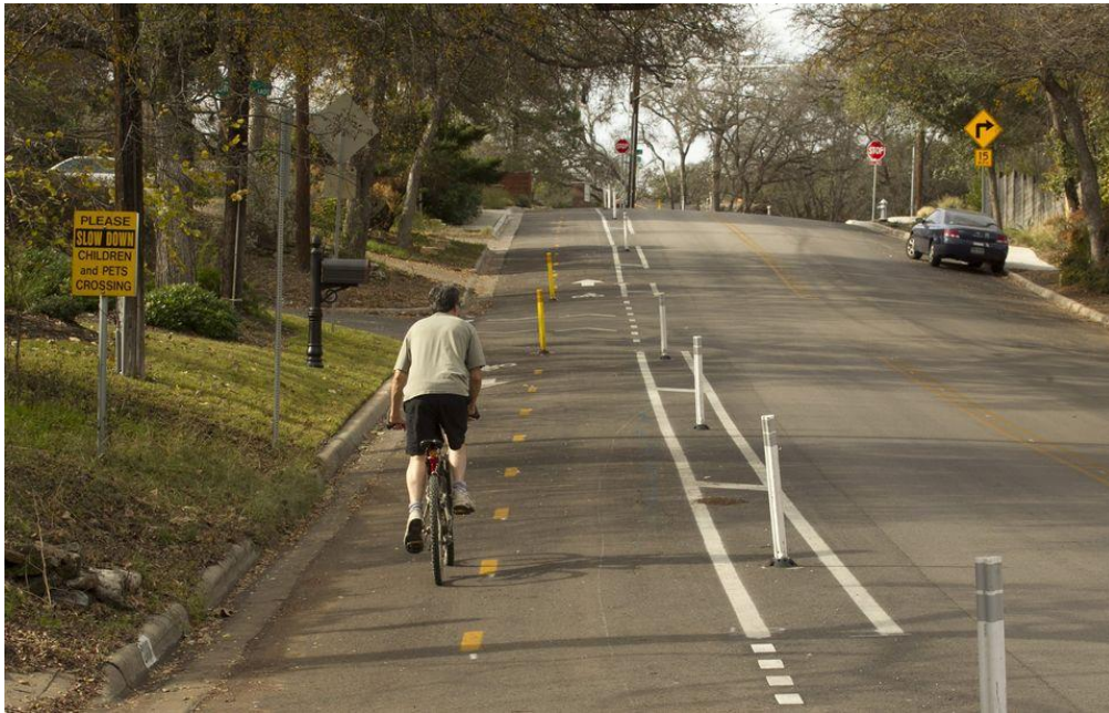
Figure 3A / Example of separated bike lane with curb and gutter cross section
