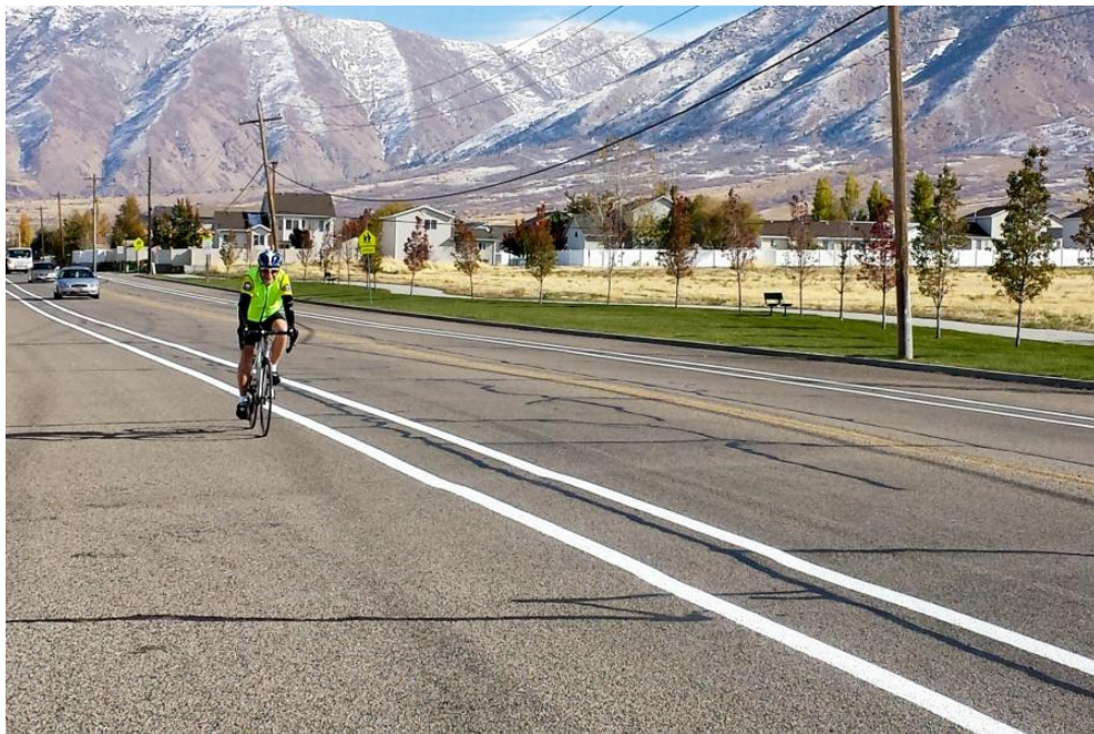
Figure 3B / Example of separated bike area with rural cross section
